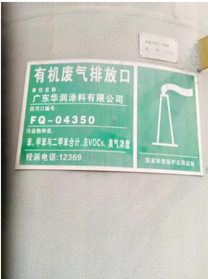
P1 废气排放口标志牌
